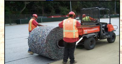
SPORTDRAIN<sub>MAX</sub> is recycled from baled waste primarily from the US automotive industry.
